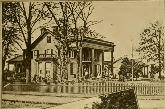
Residence of Mrs. B.B. Willis.
